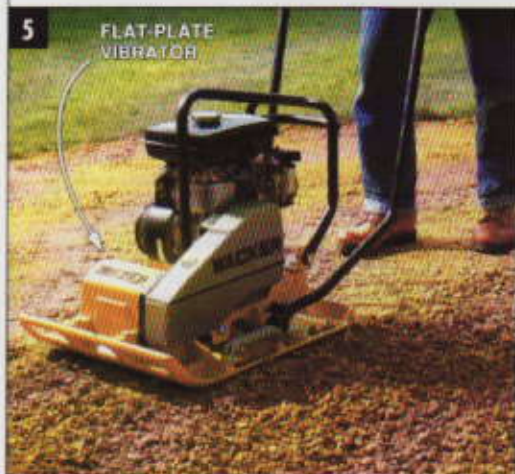
5 FLAT-PLATE VIBRATOR TAMP THE SUBBASE using a flat-plate vibrator (rented at $40 a day). Work in a circular motion and compact the area twice.
