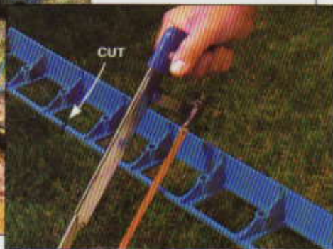
6 INSTALL THE EDGING on the tamped subbase using 8" - 10" spikes. Cut the webbing on the edging's back side to make it flex for curves.
