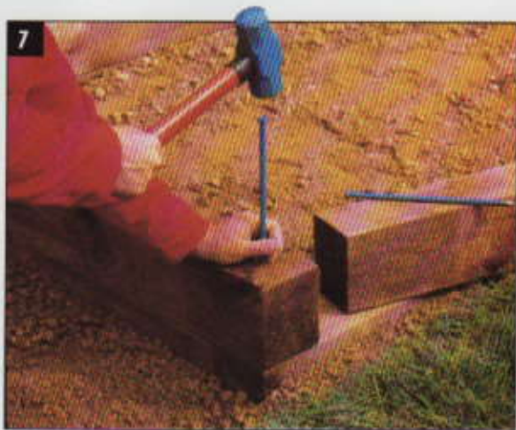
6 INSTALL THE EDGING on the tamped subbase using 8" - 10" spikes. Cut the webbing on the edging's back side to make it flex for curves.
