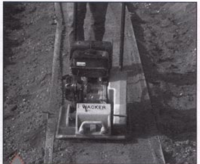
4. Compact leveling pad granular material.
