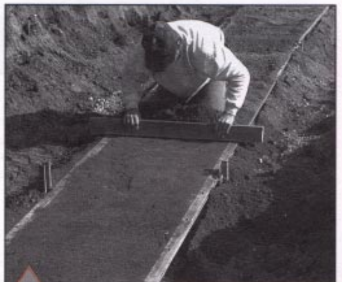
5. Screed sand for final leveling of pad.
