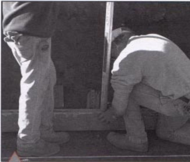
1. Set and level metal screed forms.
