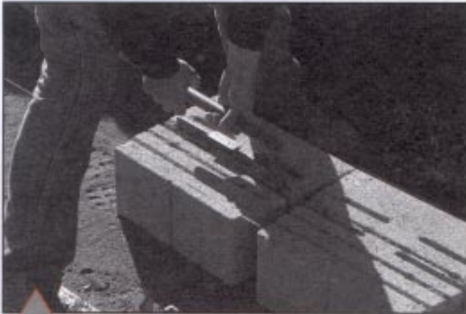
6. A VERSA-LIFTER™ aids in lifting and placing base course units.
