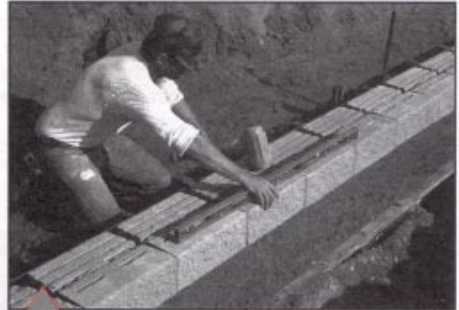
7. Use a long level to maintain consistency unit to unit.
