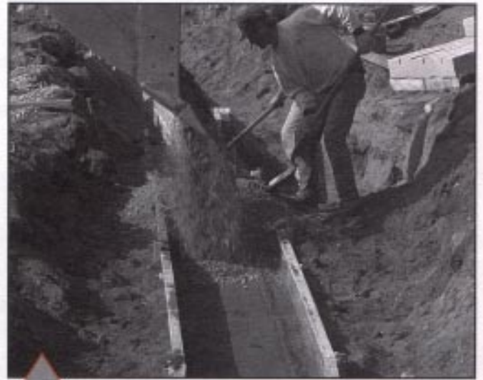
3. Fill forms with granular base material.
