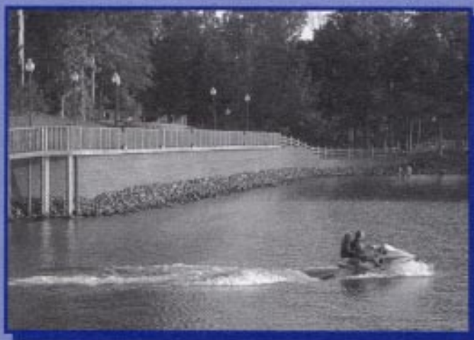
A competent foundation, protected by riprap, provides protection from continuous wave action.
