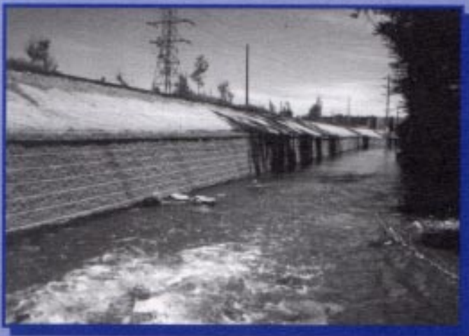
Solid, durable, interlocking SRWs are ideally suited for storm channel and flood control projects.
