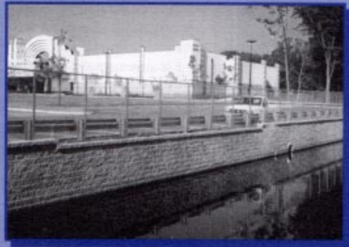
VERSA-LOK SRWs increase retention pond capacity and maximize usage of surrounding land.
